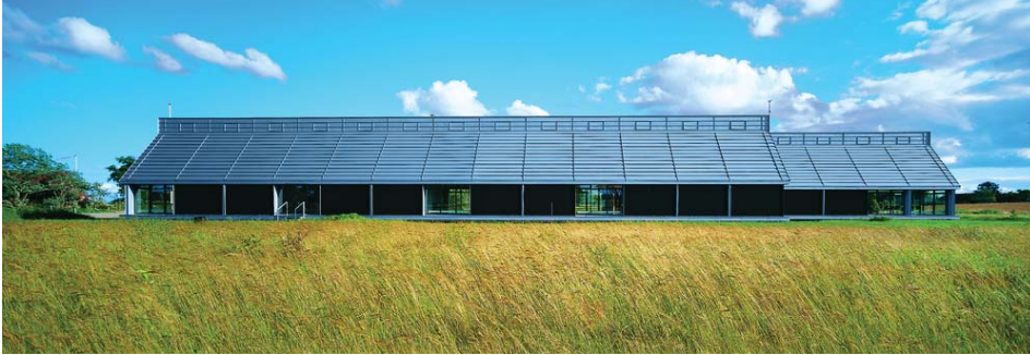
Samsø Energy Academy, Denmark
