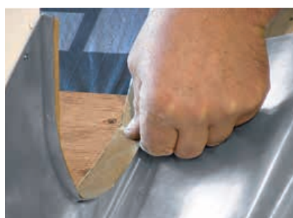
Preparing the adhesive connection
