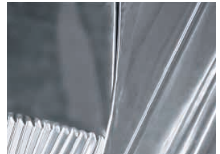
Completing the single seam
