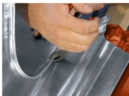
Seam preparation for back apron
