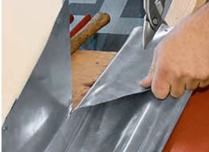
Preparing the flashing
