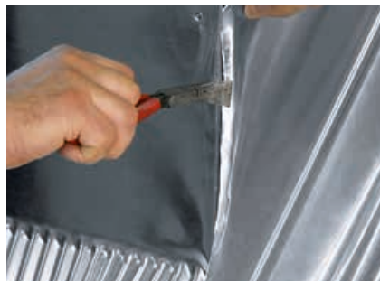
Preparing the single seam
