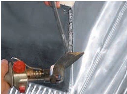
Eave-side soldering
