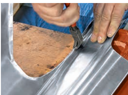
Seam preparation for side flashing
