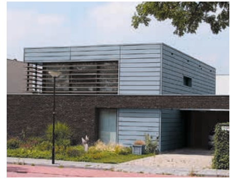
Private Residence, Empel, Netherlands
